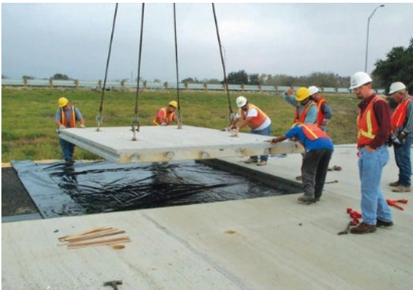
Gambar 1. Perkerasan kaku metode precast-prestressed concrete pavement .
