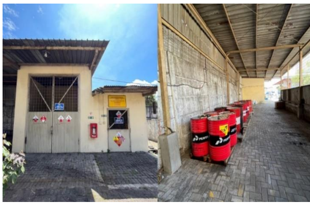
Gambar 2. (a) Tampak depan TPS LB3 (b) Tampak samping TPS LB3.
