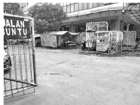
Figure 7. Physical Barrier at Zone B
