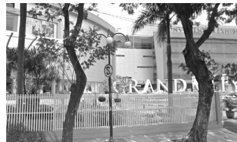
Figure 10. Physical Barrier at Zone E
